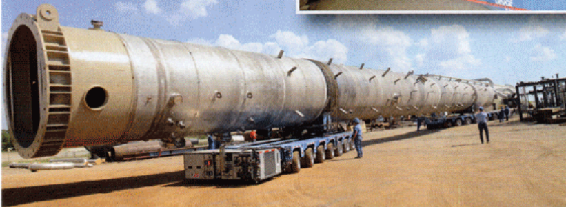
In pre-move work, Taylor's crews worked to position the trailers under the vessel.
